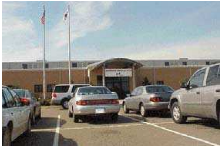
HS&AA's facility, which is the 50,000 S.F. shell building built as part of the recommendations from the economic development strategic plan. The building was financed by Alabama Power Company's speculative building program.
